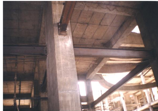
(b). Connection of steel with Concrete
