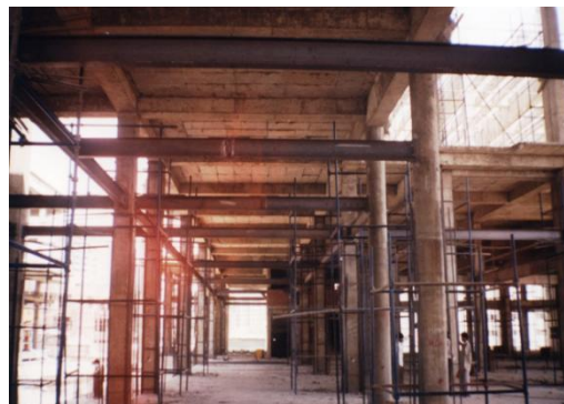
(c). Connection of steel with Concrete
