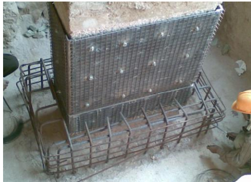
(a). Strengthening of column base
