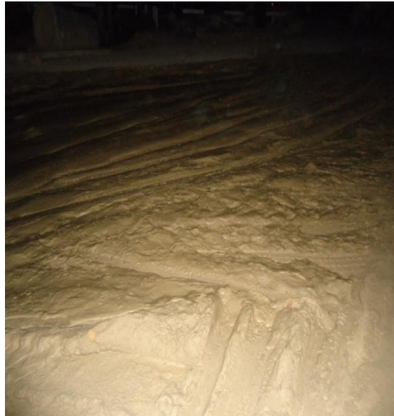
Figure 3: Road side dumping (Slippery Road)
