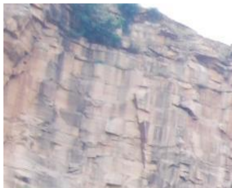
Figure 5: Joints exposed in sandstone of Vindhyan Supergroup near Golpahadia
