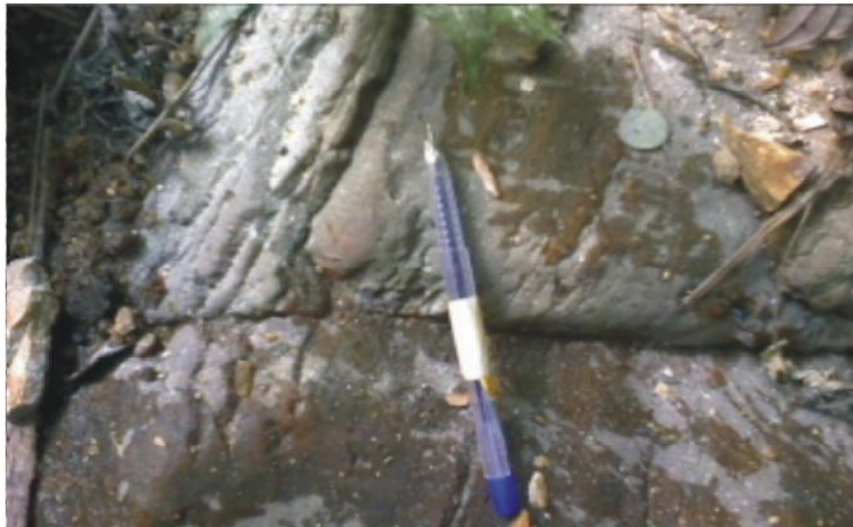
Figure 15: Fracture due to brittle nature of the rock
