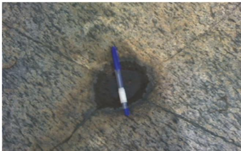
Figure 14: Solution hole caused by differential weathering
