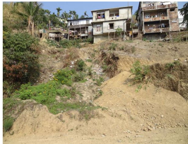
Plate 2: Areas with high slope angle coupled with unconsolidated sediments are susceptible to landslide as observed in Mamit town
