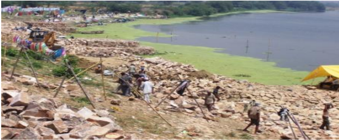
Figure 3: Photograph shows the construction work for bank stabilization on the right bank of the Gomti River near Gaughat
