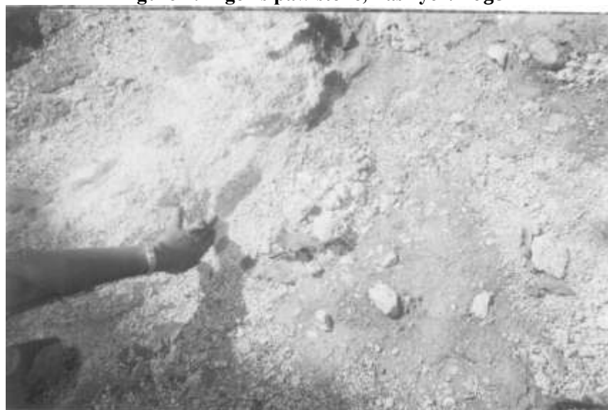
Figure 8: Granular disintegration in soda granite, Jugra village
