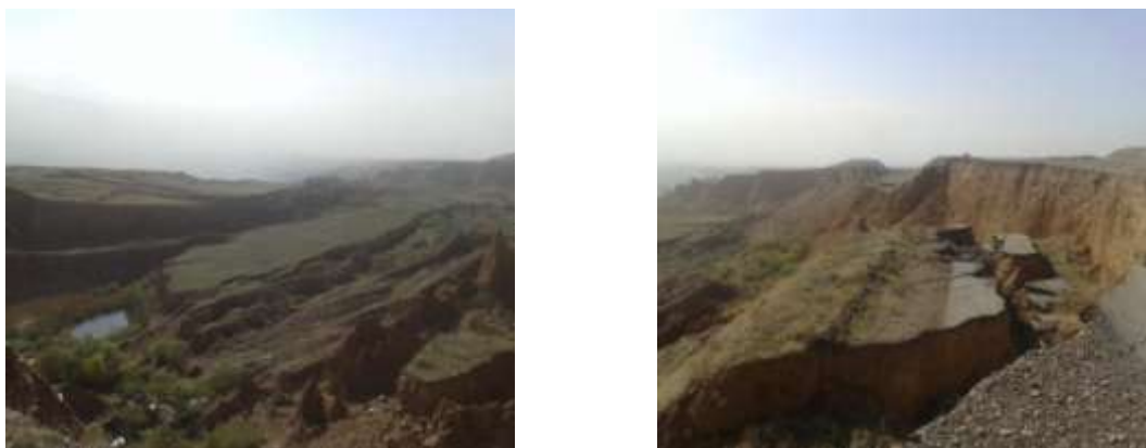
Figures 3, 4. Kokand landslide on Angren open pit
