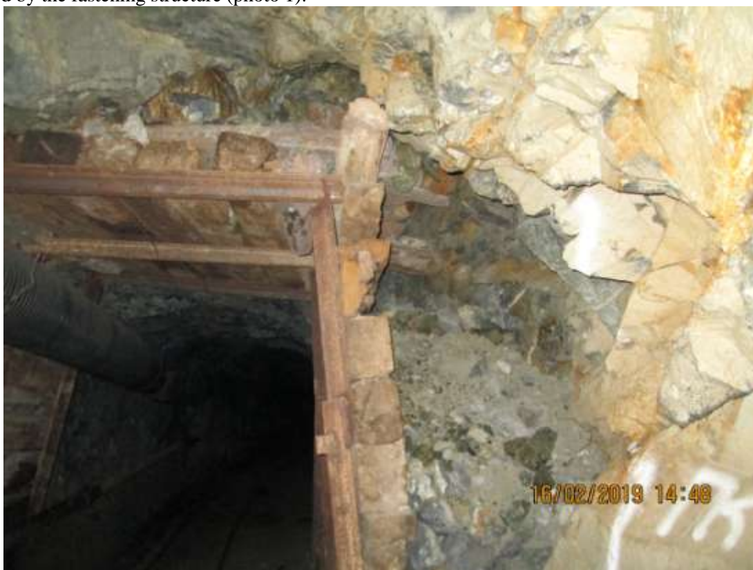
Figure 1: Dump on the roof of mine workings after sinking
