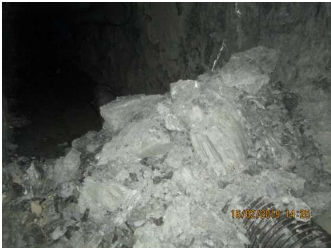
Figure 2: Caving, confined to moistened crushing zones in the right wall of mine workings
