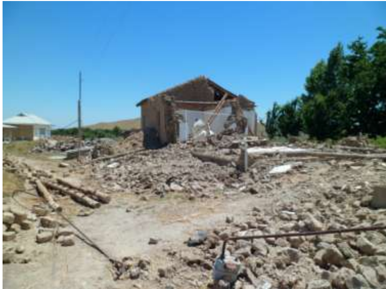
Figure 3: Damage to houses affected by the Marjonbulak earthquake of May 26, 2013 (damage level -5).
