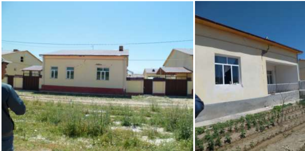
Figure 5: New type of residential buildings affected by the Marjonbulak earthquake on May 26, 2013. (damage level - 2).
