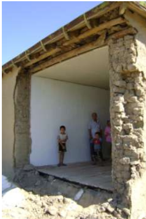
Figure 4: Damage to raw brick houses affected by the Marjonbulak earthquake on 26 May 2013. (5th and 4th damage level)
