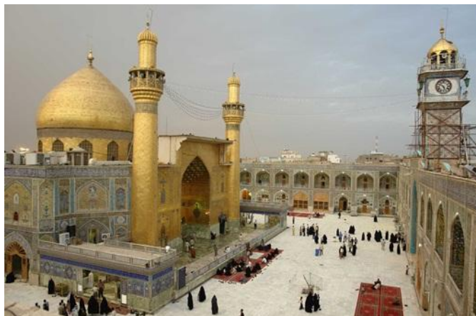
Figure 6: patios; around the yard
