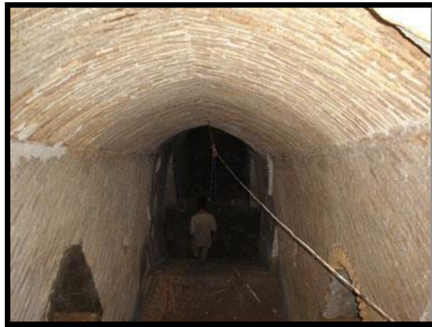
Figure 11: The Shavadun of Zargar's house. Dezfoul.
