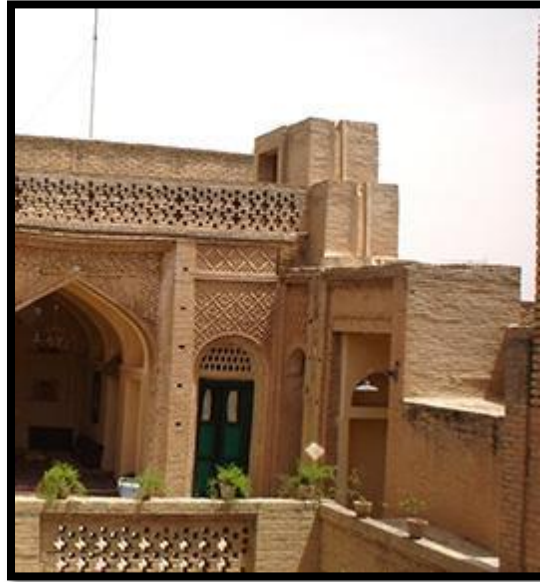
Figure 7: A view of staircase of Souzangar's House. Dezfoul.
