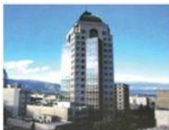
Figure 23: Armita administrative tower
