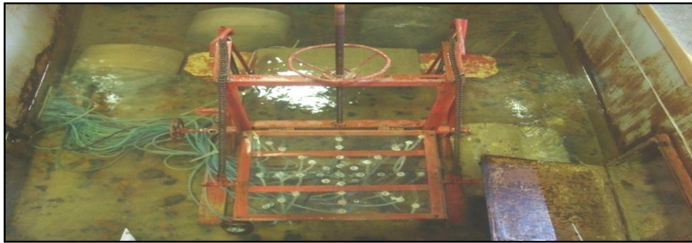
Figure 4: Jet collision sheet installed on metal system inside the jet drop storage
