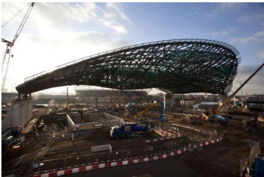
Figure 5: Use of light structures in construction of this Aquatic sport in London (Begley, 2012)
